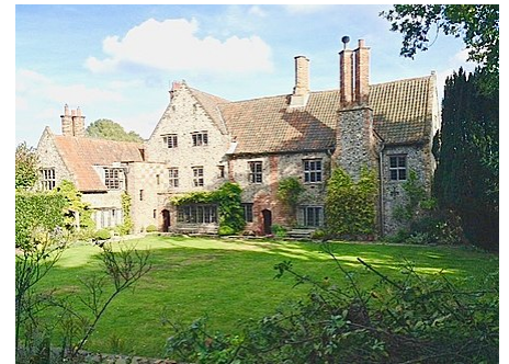
The Ivison Macadams' home Runton Old Hall, Norfolk
