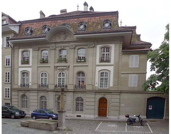
The north façade of Herrengasse 23
