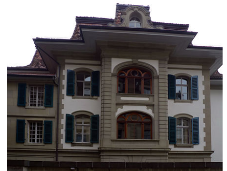
The western façade of Herrengasse 23
