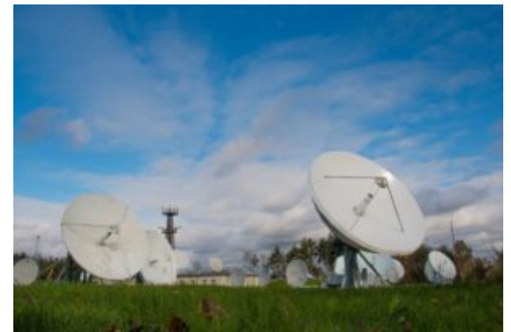
Cobbett Hill Earth Station
