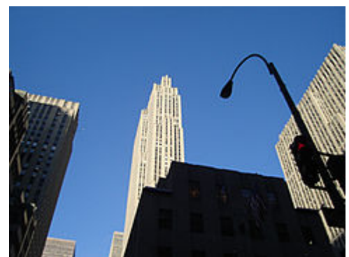
30 Rockefeller Center, also known as the GE Building, is the world headquarters of NBC.
