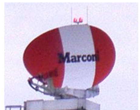
Marconi S511 radar located at Norwich International Airport
