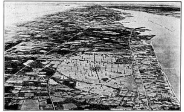
Illustration of how a fully built RCA Radio Central facility at Rocky Point, Long Island, New York would have appeared. Only two of the twelve "antenna spokes" were actually built. [11]
