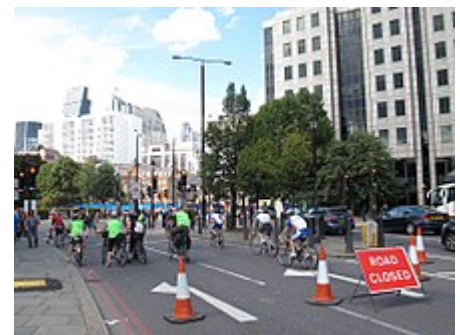
The former Hambros head office at 41 Tower Hill (on the right in the photograph)
