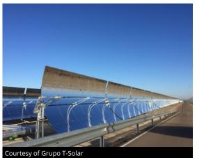
The portfolio uses parabolic trough thermosolar technology (without salt storage) and inclu 50-MW Project Moron in Seville and the 50-MW Project Olivenza in Badajoz. Since beginning operations in 2012, the two plants have delivered more than 200 GWh per year to the grid, c enough power for annual needs of approximately 160,320 people.
