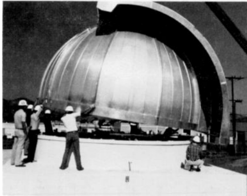
Optical domes being installed at GEODSS Test Site.
