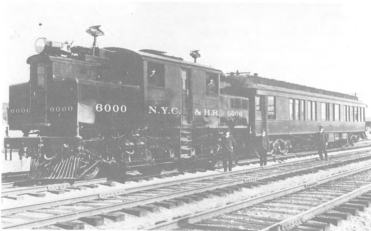
Ninety-four-ton gearless electric locomotives for the New York Central Railroad.
