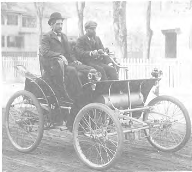
The "Uniflow" engine steam carriage developed by Thomson and Lemp.
