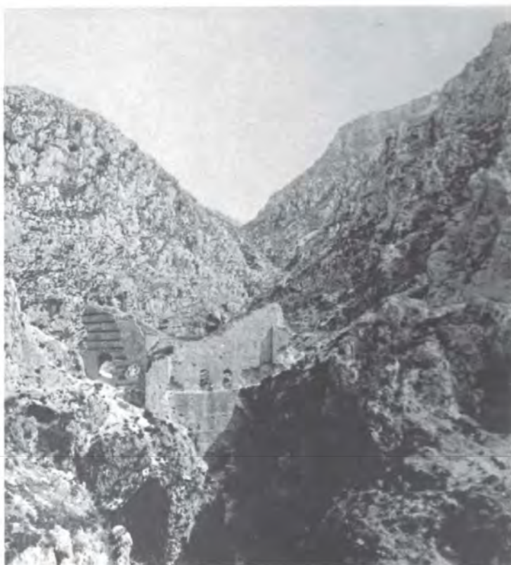
17. "IRON GATE" (BAB EL-HADID), 1934, looking east, from within the city. The masonry is of the time of Justinian. The structure, described by Procopius, was designed to control the torrent that entered the city here. The city wall, in which the Gate stood, has disappeared at this point. (Photograph courtesy of the Committee for the Excavation of Antioch and its Vicinity.)
