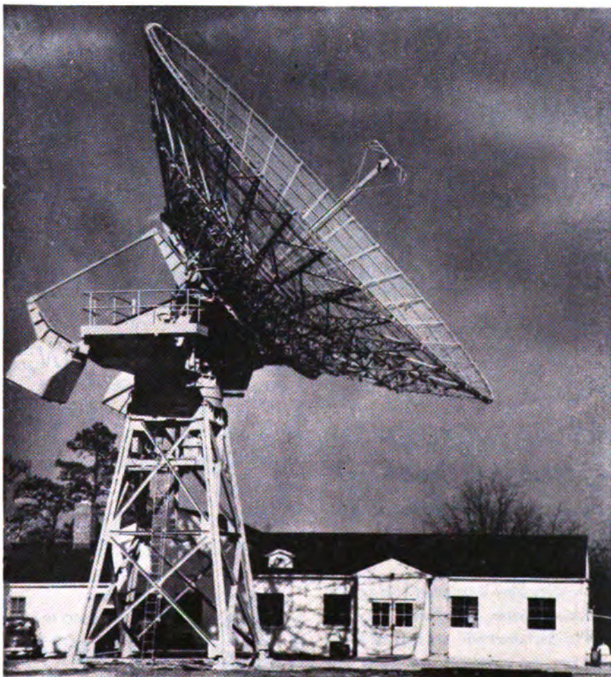
Shown above is the assembly of antenna, mount and tower of the Diana Radar System for use in very long-range radio propagation
