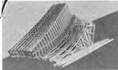
28 ft. antenna knocked down for air freight shipment
