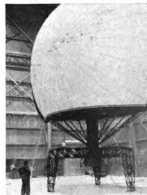
The 30-foot antenna shown here, ready for operation, weighs only 1690 pounds complete with its base and tripod. It will rotate at 6rpm driven by a ¼-hp motor.
