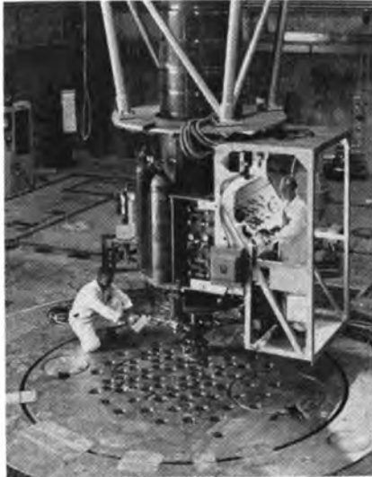
A huge, lead-shielded chamber for loading uranium fuel into the atomic energy reactor hovers over the "core" or heart of the reactor sunk deep beneath the ground. Heat from the atomic "furnace" is used by the experimental power station to generate electricity.
