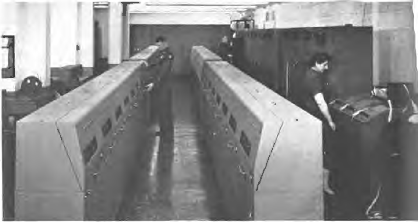
Overall view of the Switching Center
