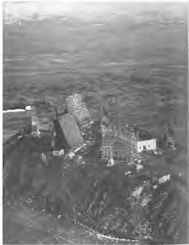
Completed station (above left) in Matanuska Valley area interconnecting tropospheric scatter path and microwave radio path. Scatter station (above right) interconnects three paths with two antennas for each path. Two paths require 60 ft. rectangular parabolic antennas, and one uses a 30 ft. circular parabolic antenna.
