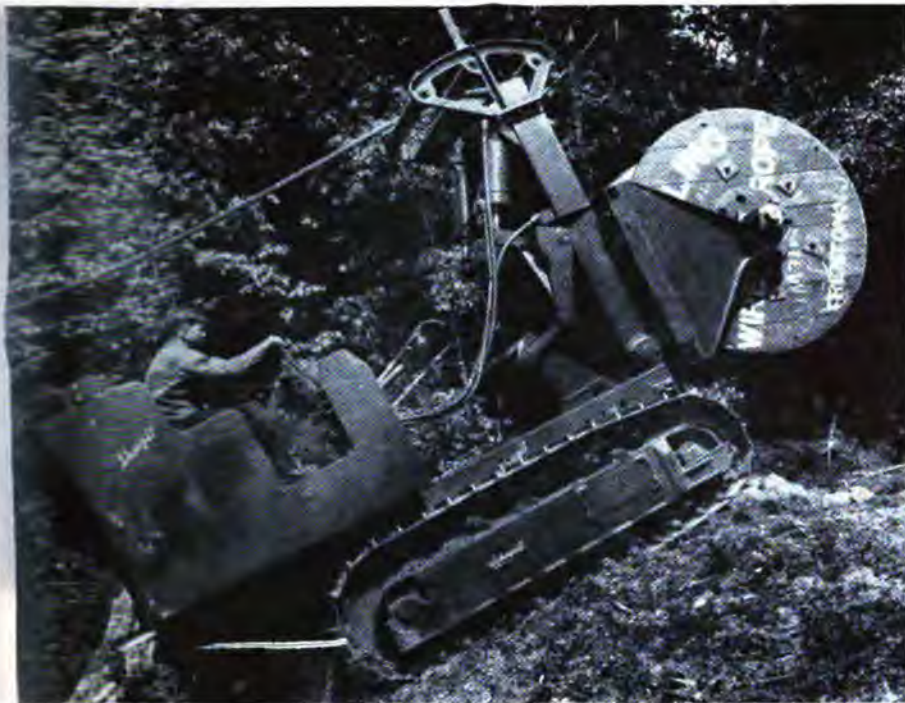
In going up hills, the load is thrust far forward to provide maximum traction. Lift carriage is vertical. Note fairleads for paying out cable when machine moves forward.
