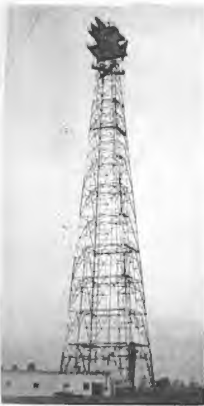
At certain interconnection points along both the express and by-pass routes, radio relay main stations like the one pictured here, will tie the new routes into the network.
