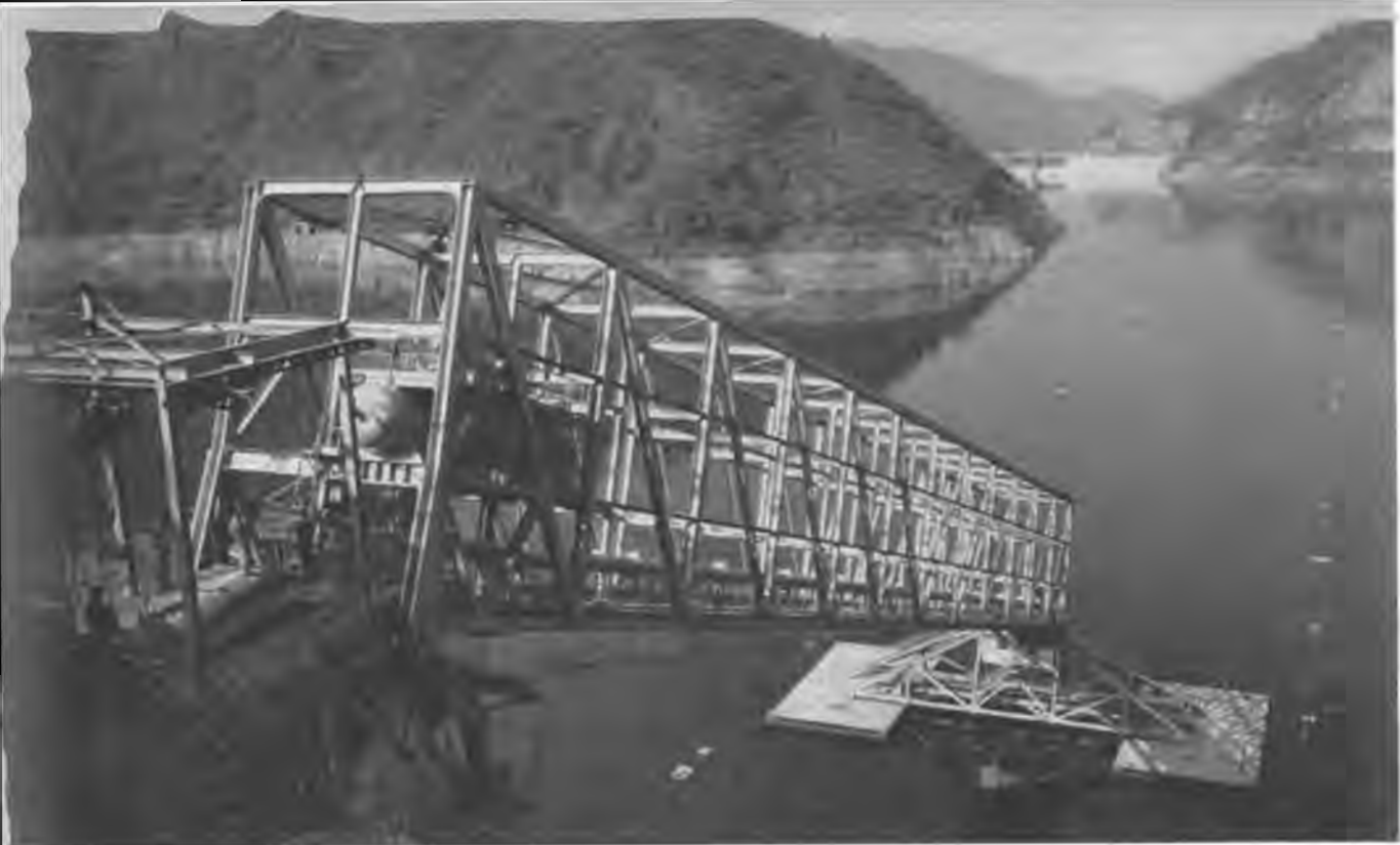
The Variable Angle Launcher, one of NOTS' test facilities, is considered the largest "blow-gun" in the world. Experimental missiles are blown into the water through a 300-foot long launching tube.
