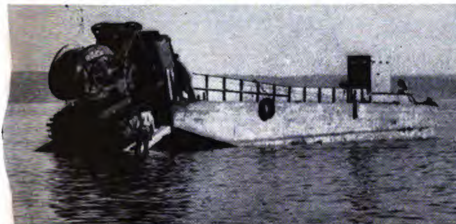
Trac-Karrier ran in four feet of salt water, laying and picking up cable to and from landing craft. Note the load pulled back over the tracks as it backs up ramp.
