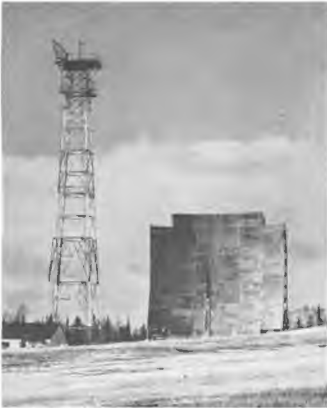
Completed station (above left) in Matanuska Valley area interconnecting tropospheric scatter path and microwave radio path. Scatter station (above right) interconnects three paths with two antennas for each path. Two paths require 60 ft. rectangular parabolic antennas, and one uses a 30 ft. circular parabolic antenna.
