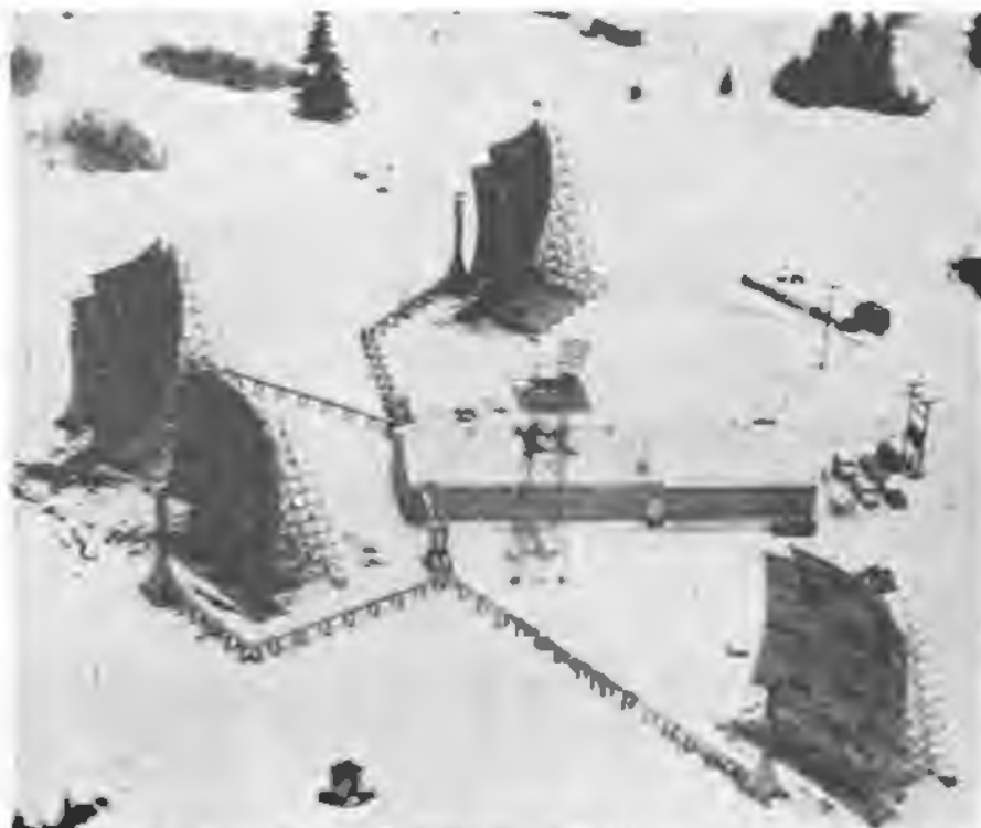
A completed station in the White Alice communications system on the Kenai Peninsula interconnecting two tropospheric scatter paths and one microwave radio relay path.
