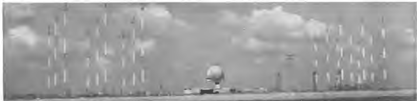
Corner reflectors used in rearward communications
