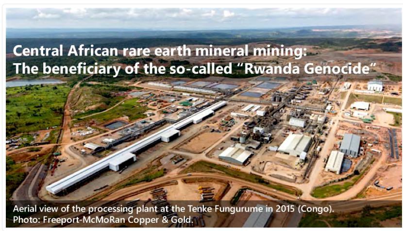
Fig. 2—Aerial view of the processing plant at the Tenke Fungurume in 2015 (Congo). Photo: Freeport-McMoRan Copper & Gold.
